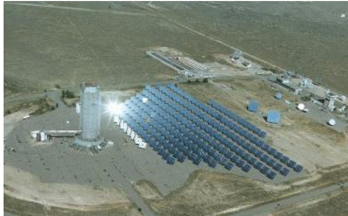
Figure 1: Sandia National Laboratories National Solar Thermal Test Facility heliostat array. This array consists of 222 heliostats and a single 200ft tall power tower.
