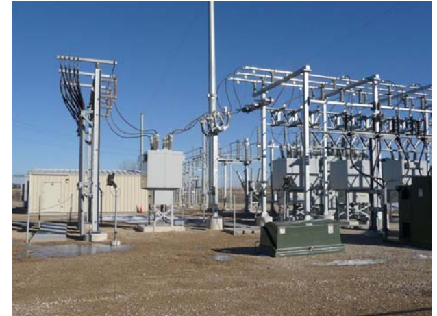
Collection Bus Breaker & Substation Bus
