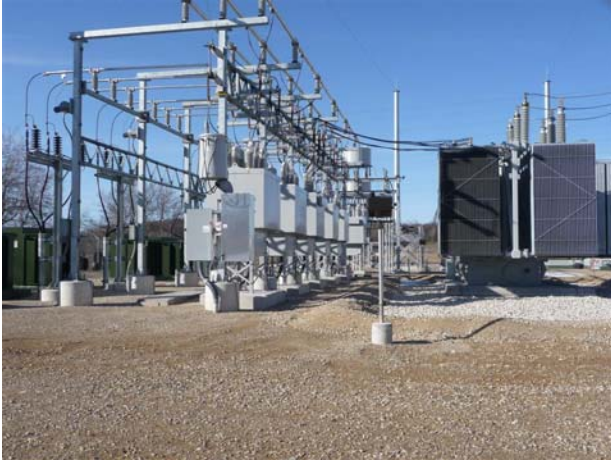
Collector Breakers & Transformers
